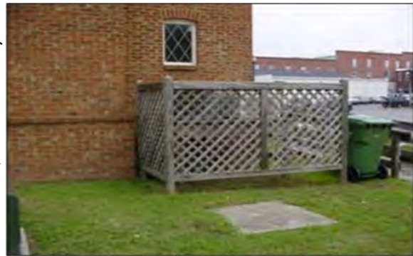
Mechanical systems should be screened from view.
